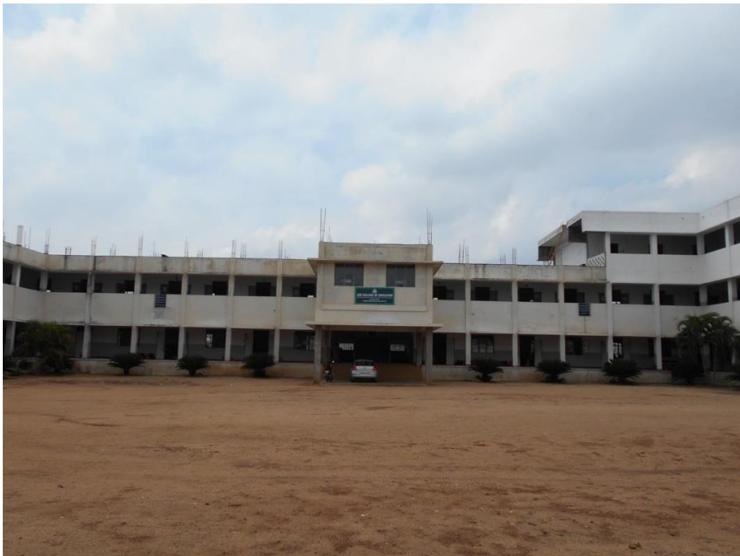
18. Open Space for Additional Accommodation JSR COLLEGE OF EDUCATION (10316) Madathukulam (PO & TK), Tiruppur DT – 642 113.
